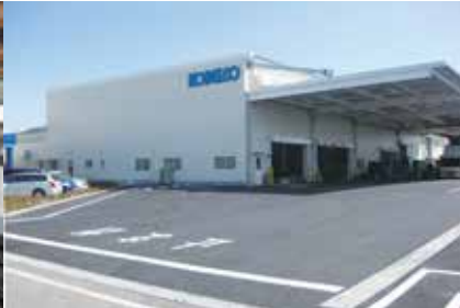
Ogaki Factory, birthplace of our hydraulic mini excavators
