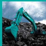
Aggregate processing and material sorting
