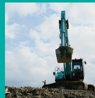
Rubble receiving and aggregate processing
