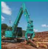
Timber transport and handling
