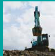
Rubble receiving and aggregate processing
